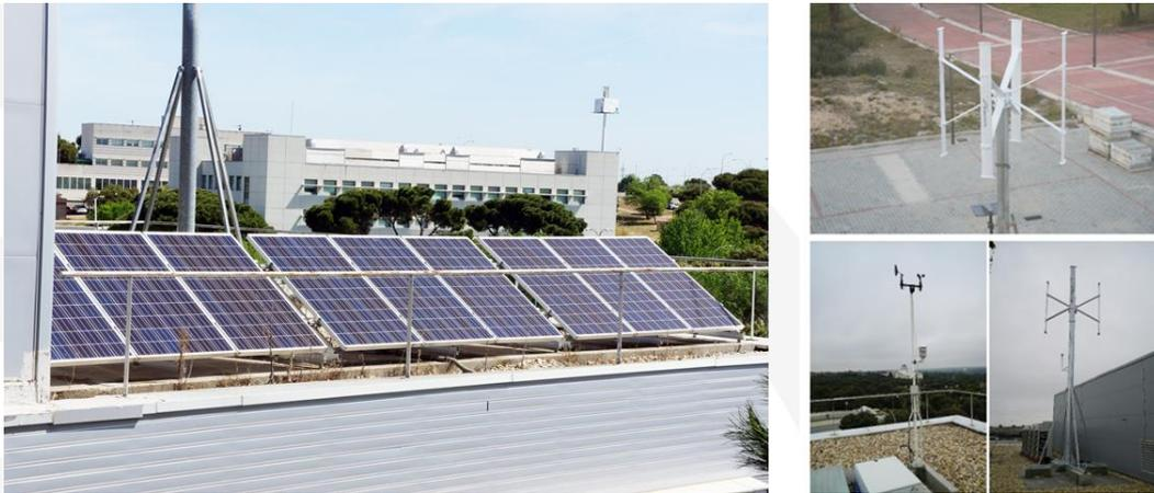
Fig. 12. Microgrid located at the rooftop of CEDINT-UPM: PV panels (left) and wind turbines (right).
