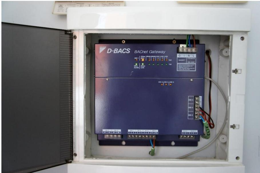
Fig. 13. HVAC control system that allows the communication with HVAC indoor units.
