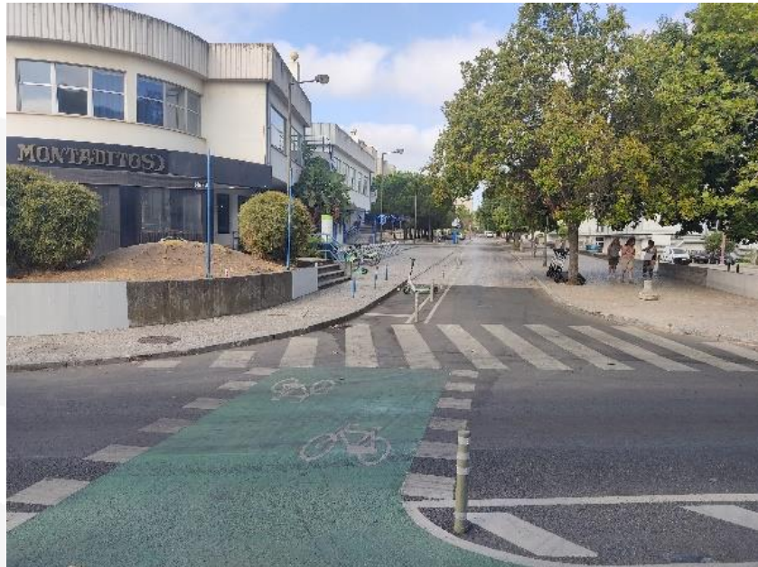
Figure 2 – Eastern entrance of Access 1
