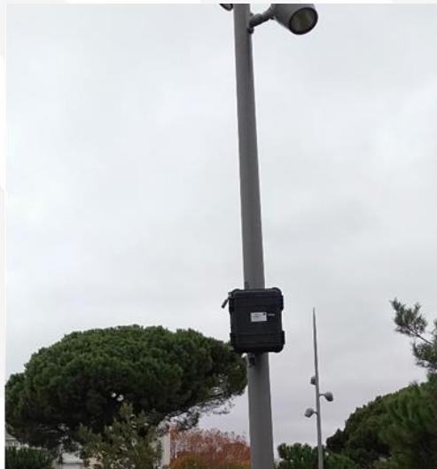
Photo 2. Trafficradar: motor vehicles
