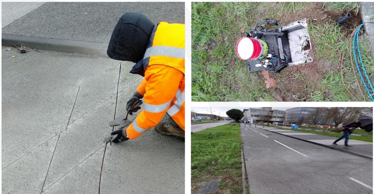
Photo 4: Installation of the ZELT loop: bicycle counter
