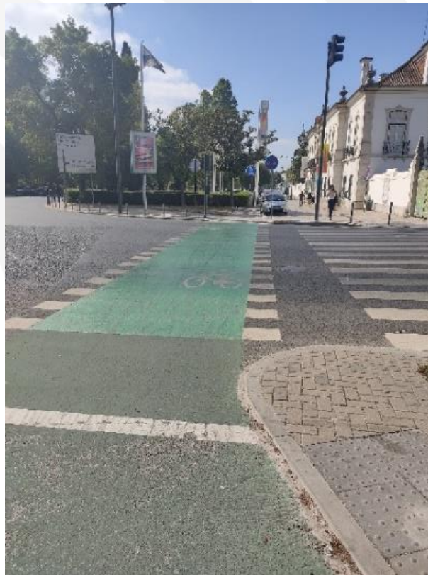
Figure 4 – Pedestrian and cycle path leading to Access 3
