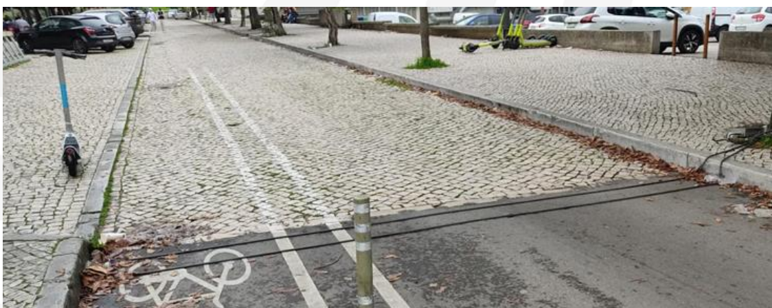
Figure 7 – Pneumatic tubes, which allows the detection of the passage of bicycles and e- scooters, installed at Access 1
